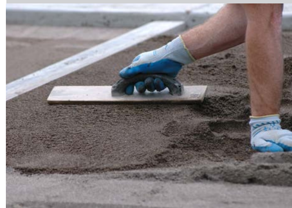
Utilize all engineering controls and PPE!
