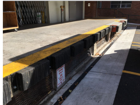
Pay attention to surroundings and keep a safe distance from dock edges!
