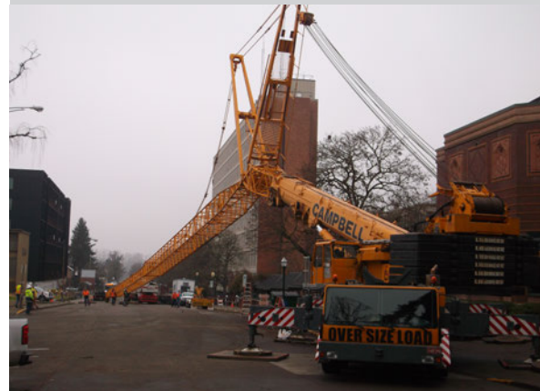
Ensure all outriggers are in place before crane setup!
