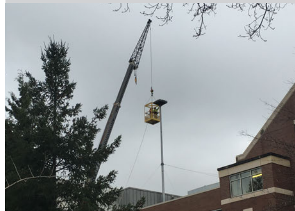
Do not exceed the crane’s load capacity!
