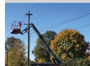
Stay at least 10 feet back from power lines!
