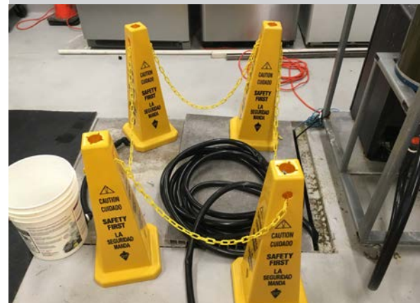
Properly guard the entrance of the space for duration of work!
