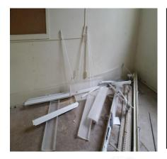
The left is an example of improper handling of Universal waste. The bulbs are not boxed and not protected from breakage. Boxes must be labeled/dated, in good condition and sealed.
