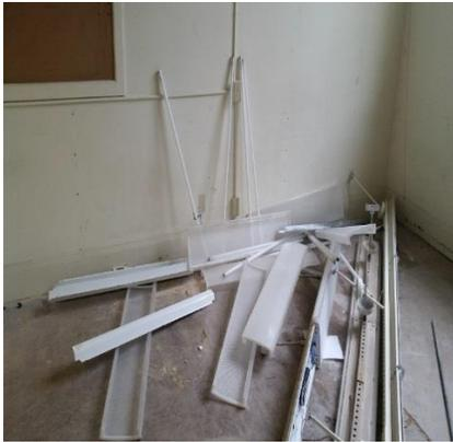
The left is an example of improper handling of Universal waste. The bulbs are not boxed and not protected from breakage. Boxes must be labeled/dated, in good condition and sealed.
