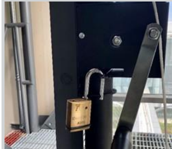
Always realign the tabs and replace the lock before climbing
