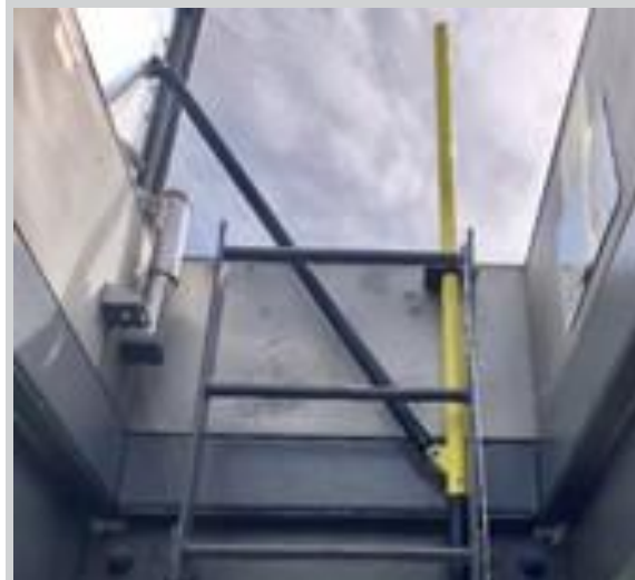
Use the pop-up bar to help you move from ladder to roof and back.
